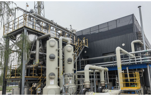
After retrofitting: Alkali spray absorption + Water spray absorption + Resin adsorption
